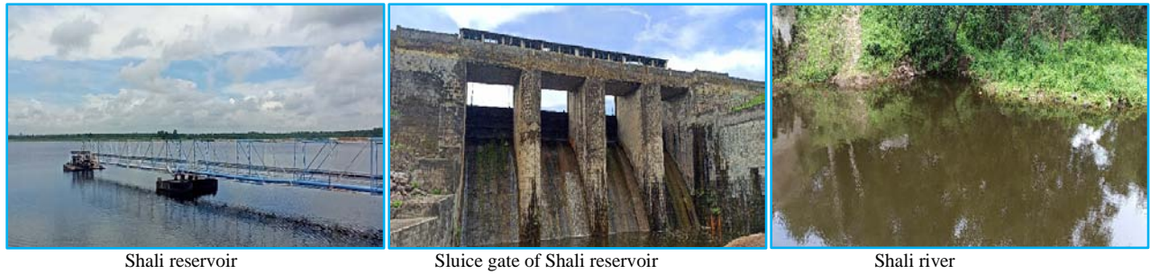
Fig. 2. Images of the Shali reservoir system, taken during the field visit
