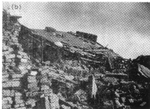
Fig. 3(b). A double storeyed building collapsed at Chapra, killing five persons
