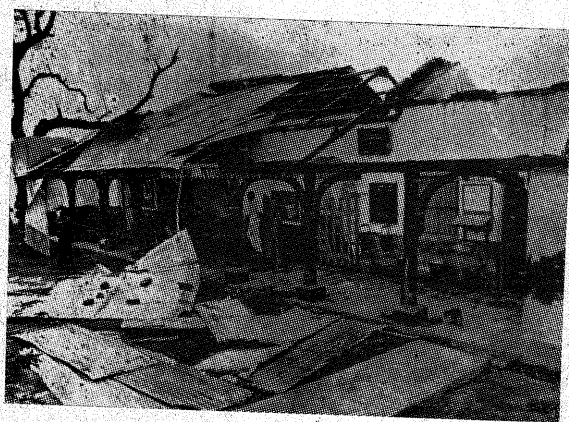
Fig. 5. Tettu railway station in Prakasam district damaged by May cyclone
