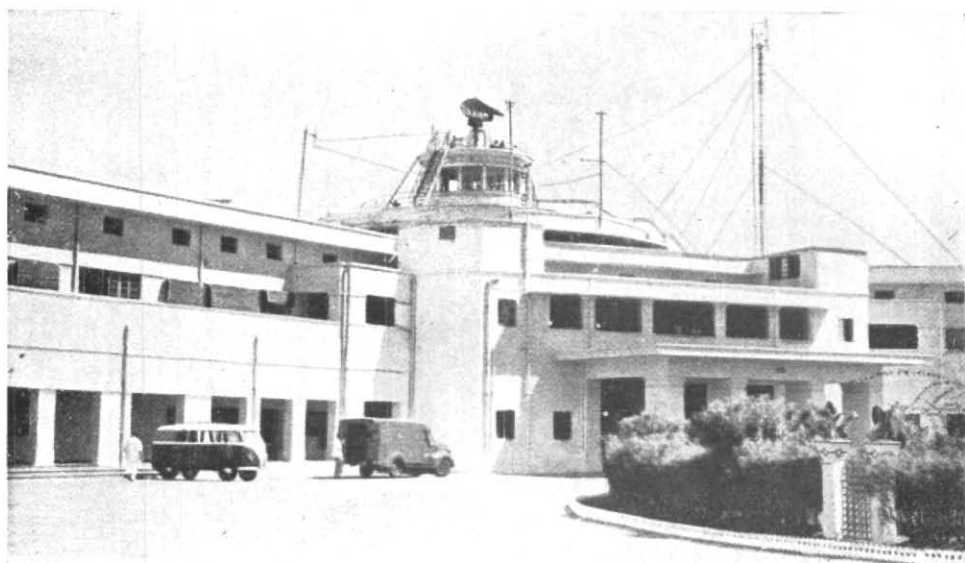
Fig. 1. Photograph of the scanner unit on the top of the Control Tower of the terminal building at Meenambakkam Airport, Madras
