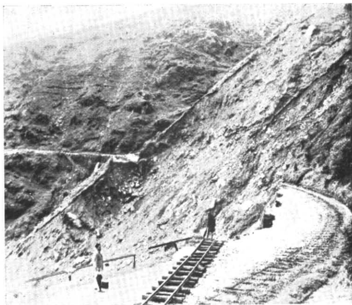
Fig. 2 One of the major landslides which uprooted the railway line between Darjeeling and Kurseong (Photo : Amrita Bazar Patrika, Calcutta )
