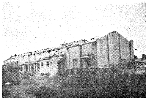
Fig. 5. View of barrack No. 197 from the northwest
