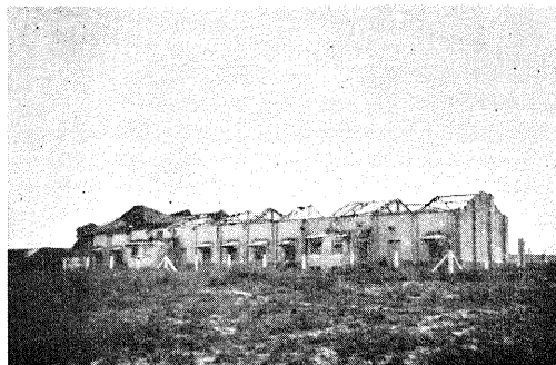
Fig. 3. View of barrack No. 199 from the north
