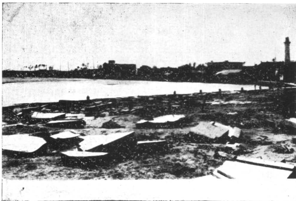
Fig. 3. Nagapattinam port wall lies broken and scattered on the beach (Photo : The Hindu, Madras )
