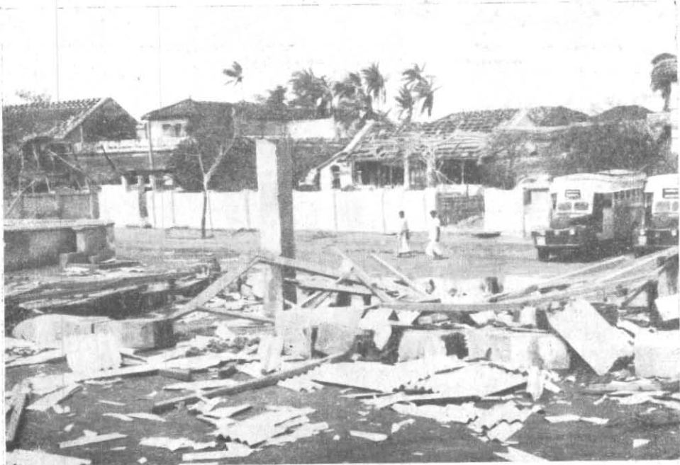
Fig. 2. The damaged municipal bus stand at Nagapattinam (Photo : The Hindu, Madras )
