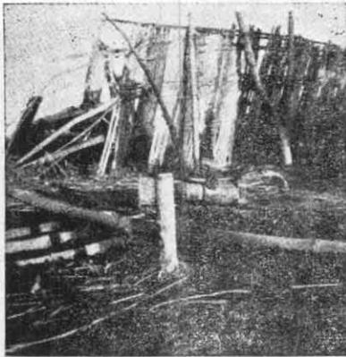
Fig. 7. The pump of a tube-well broken off from the main tube which was thrown off nearly 30 metres away. The pump is picked up and placed near the main tube for taking photograph
