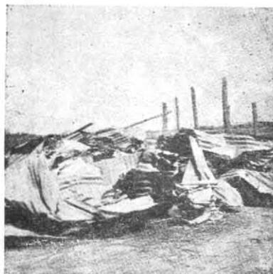
**Fig. 3.** Torn-off and twisted C. I. sheets blown off to distant places were collected and kept together after the tornado was over
