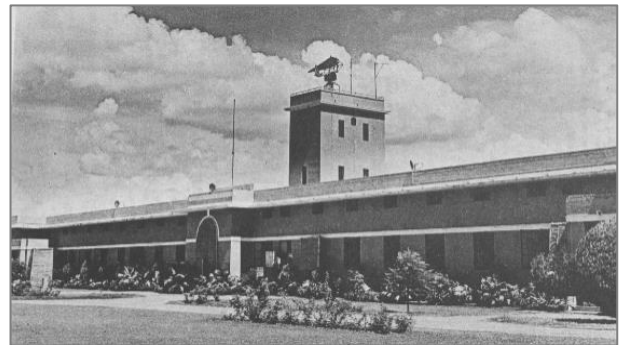
Fig. 3(b). "Aerological Offices and Observatory", IMD's headquarters in New Delhi, 1944-1975
