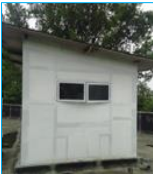
Fig. 52. Radiation calibration hut
